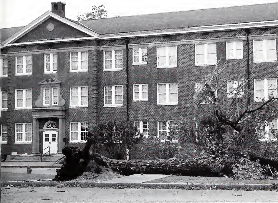
Left: The front of Mobile Hall.
